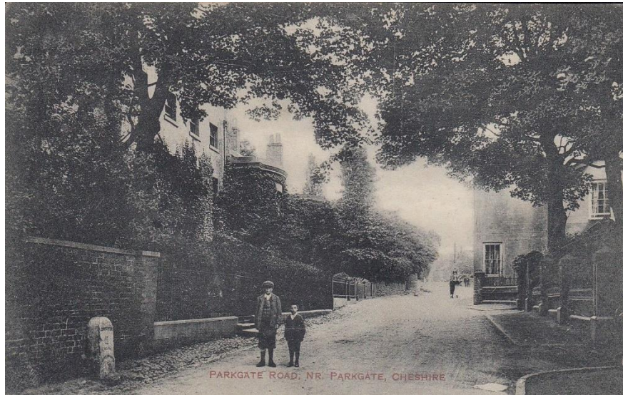
Parkgate Road c 1908, with the 'Chester 11 miles' stone of 1787 still in place
