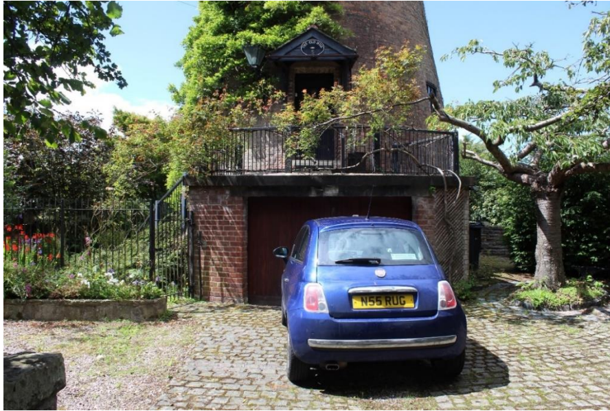
Neston Mill now a home – July 2020 Photo: Alan Passmore
