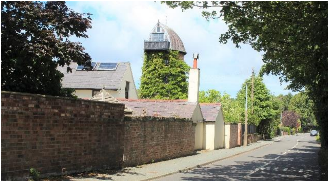
Neston Mill and Mill Cottage in July 2020 Photo: Alan Passmore
